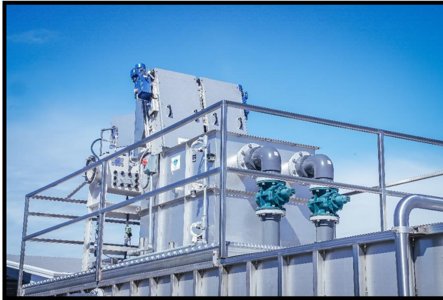
Example Duplex Screen arrangement (not project specific).
